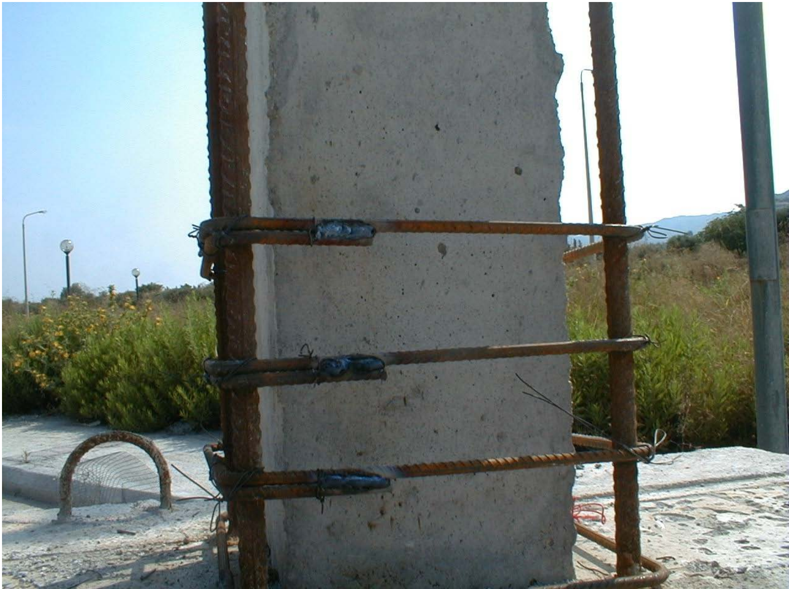
Welding of jacket's stirrup ends
