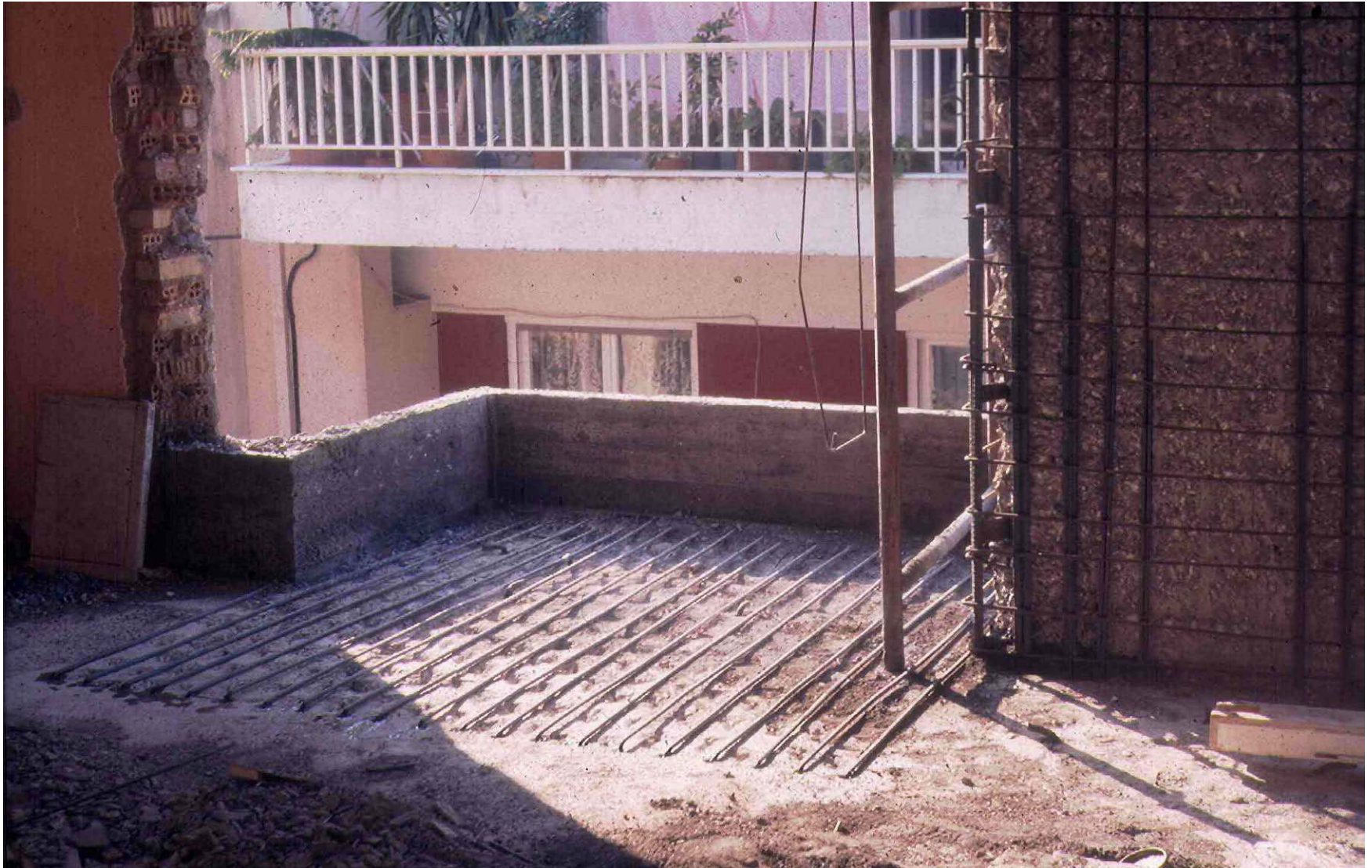
Addition of a new concrete layer to the top of a cantilever slab
