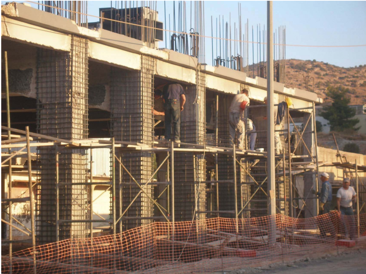
Concrete jacketing in practice
